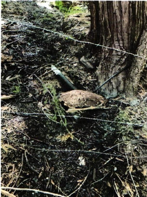
Figure 1. 1602(a) violation includes substantial diversion of the natural flow of an unnamed tributary to Lamb Creek. The screen box was the intake for POD 1 while the corrugated plastic pipe collected flow and directed it to the intake. The black poly pipe was supplemental water diverted from POD 2.
