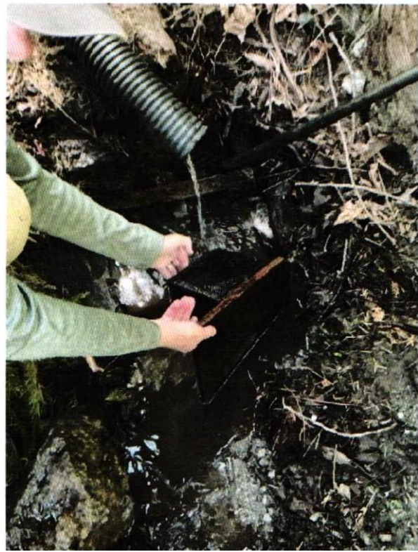
Figure 1. 1602(a) violation includes substantial diversion of the natural flow of an unnamed tributary to Lamb Creek. The screen box was the intake for POD 1 while the corrugated plastic pipe collected flow and directed it to the intake. The black poly pipe was supplemental water diverted from POD 2.
